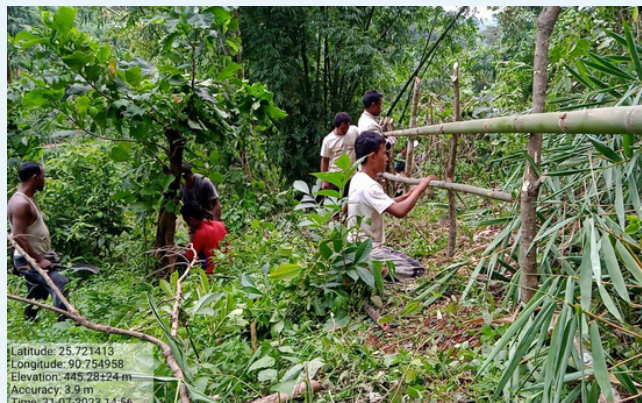
Completion of fencing at Mejlgre Nokat village.
