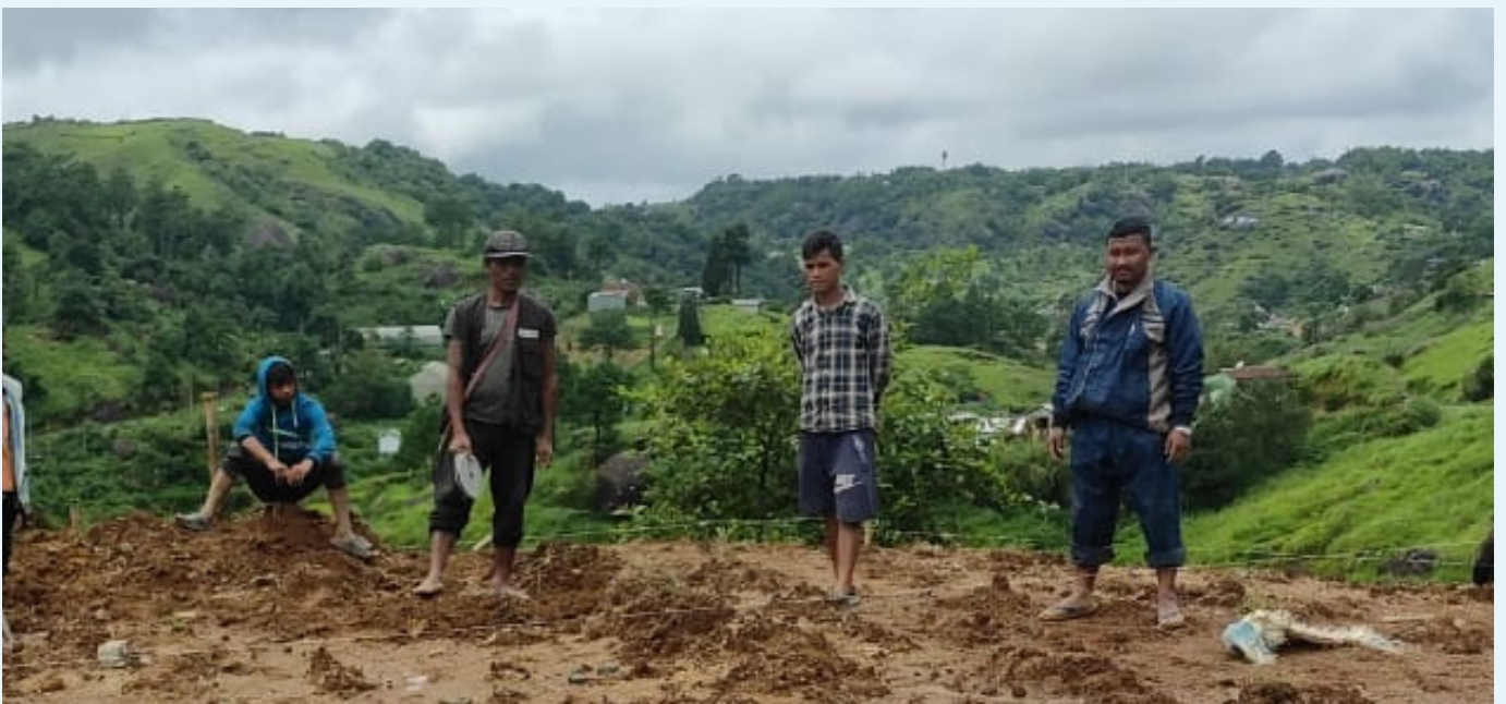
Alignment of column footing at Mawkyllung village.
