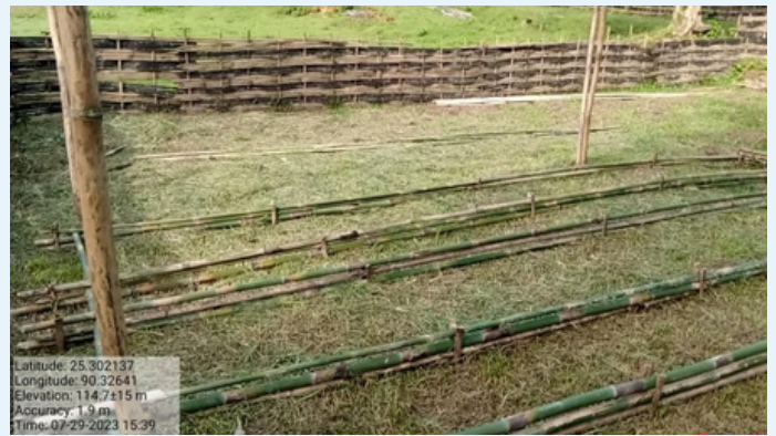
Nursery extension work at Galwanggitok VPIC.
